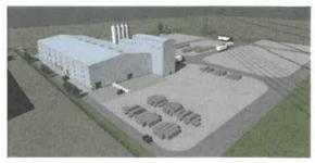
The 4.000 m<sup>2</sup> production hall will be built on a 40.000 m<sup>2</sup> site where the latest developed German machinery line will be installed for the production of 800.000 m<sup>2</sup> of paving stone per year.
